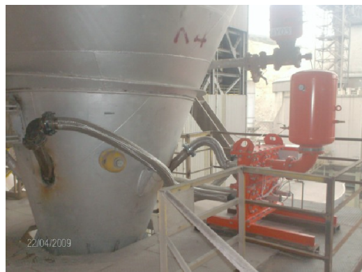
Meal Pipe Cyclone Discharge.
