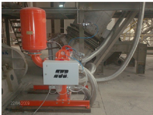
Keeping components centralized allows for easier and safer service.
