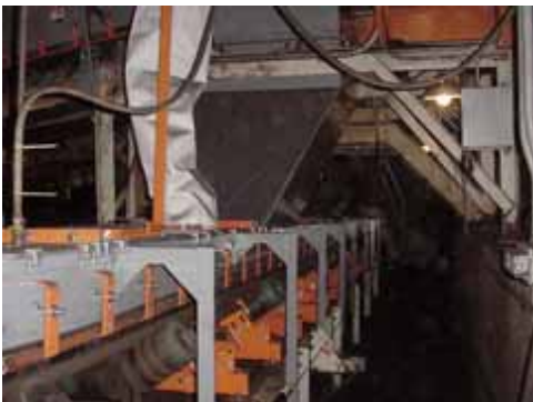
Included in the coal-conveying system reconstruction was the installation of Martin® ApronSeal™ Skirting and Martin® Dust Bag.
