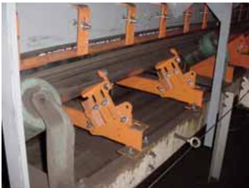
Martin® Support Cradles were installed to stabilize the belt path and reduce spillage.
