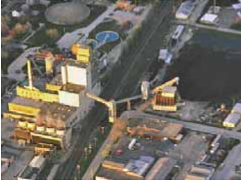
The City of Ames Power Plant burns 270,000 tons of coal per year.
