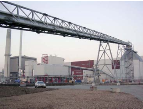
Able to power up to 600 feet (183 meters) of belt with a single low-power fan
