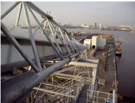
To accommodate space limitations at the Emden facility, the conveyor structure was engineered with an innovative triangular framework
