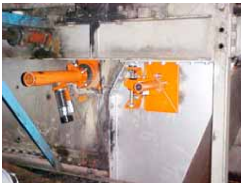
Belt cleaners from Martin Engineering are installed in the new dribble chute at the Consumers Energy D.E. Karn Plant.
