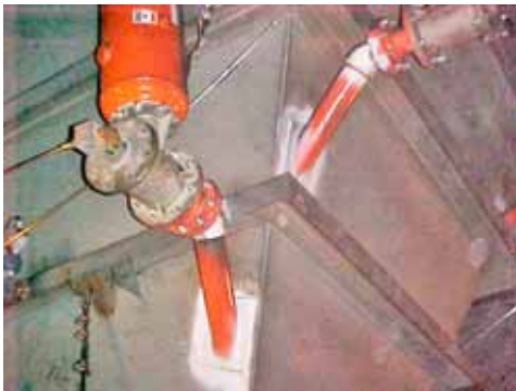
The air cannons are installed to discharge down each hopper's valley angles to clear material from the vessel.
