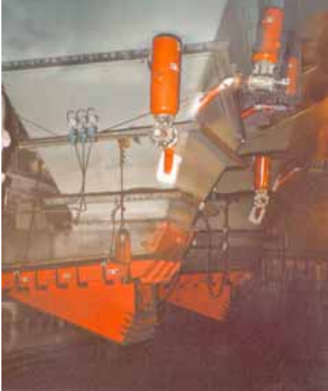
At the US Steel PCI operation, a group of six air cannons was installed on each of the three feed hoppers below the railcar dump.
