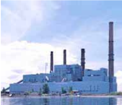
Brayton Point Station
