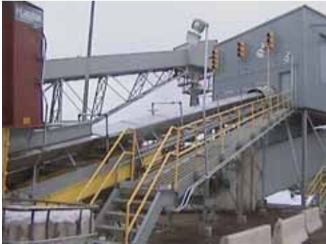
The Martin® Air Supported Conveyor at Colorado Springs Utilities, Martin Drake Plant is 60 feet (18.3 m) in length.
