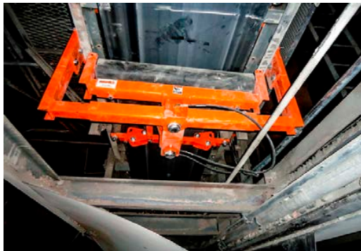
Each conveyor was fitted with a Martin® Tracker™ for the return side, to help reduce edge damage, prevent spillage and extend belt life.
