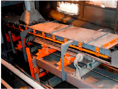
Each transfer point received one new impact cradle and two belt support cradles.
