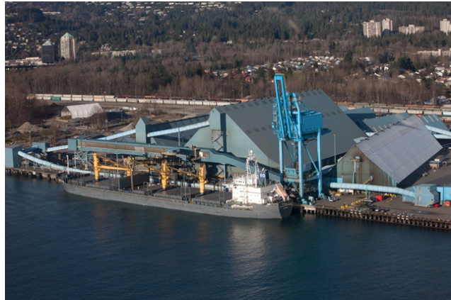
Martin Engineering designed and installed six new conveyors at the Vancouver Wharves Kinder Morgan terminal, ranging from 105 feet (~32 meters) to 709 feet (216 meters) in length.
