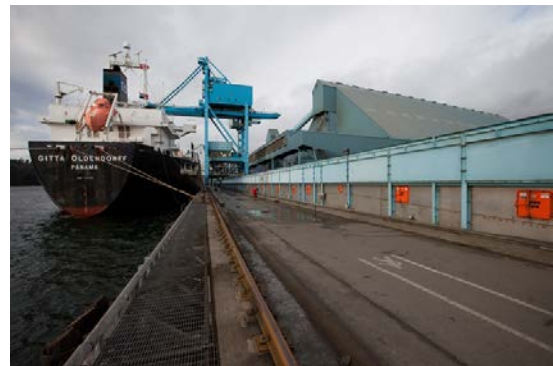
At the terminal all the minerals concentrate storage and handling facilities are fully enclosed to ensure no mineral concentrate escapes into the environment or migrates into the ocean.
