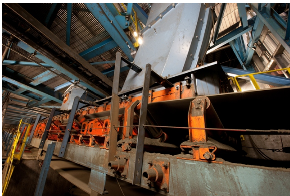
Four of the new transfer points employ a "hood and spoon" transfer, with the hood discharge chute at the top of the system and a spoon receiving chute to place material onto the belt being loaded.
