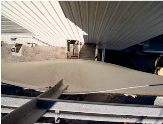
The severity of the material build-up became apparent to system operators when they noticed the walls of the silos starting to bulge outward from over-pressurization.
