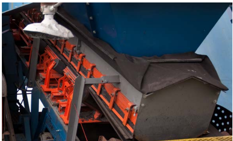
With the new conveyor Load Zone from Martin Engineering, the terminal has increased the average load rate for the entire ship-loading process from 700 mt/h to 858 mt/h.
