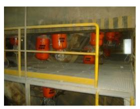
[Izmir, Turkey] — A leading Turkish cement producer has specified high-performance air cannons to replace an under-performing existing system, which was jeopardizing the plant's output capacity by failing to remove accumulated material from the preheaters. The new air cannon network resolves build-up issues that previously needed manual removal on a daily
