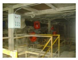
exit nozzle that's installed through the wall of the vessel or duct. In addition, the improved air path of the Tornado fills the reservoir 3-4 times faster than standard cannons.
