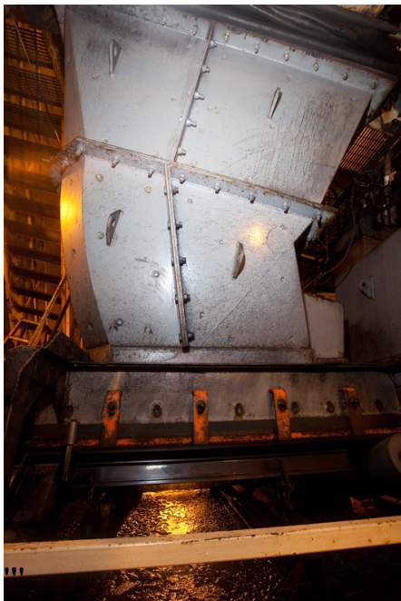
The high-efficiency insertable air cleaner is a self-cleaning design with filter elements approx. one-eighth the size of conventional filter envelopes.
