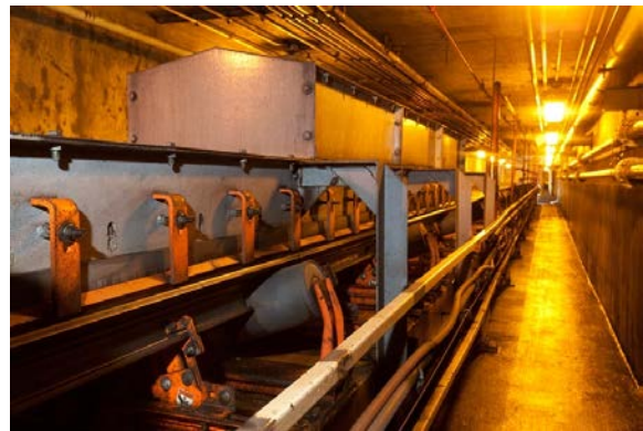
The new support system under the skirt board better supports the edges of the belt and helps eliminate sagging.
