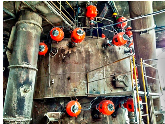
Installed in a series sequenced for maximum effect, the air cannon network is timed to suit specific process conditions.
