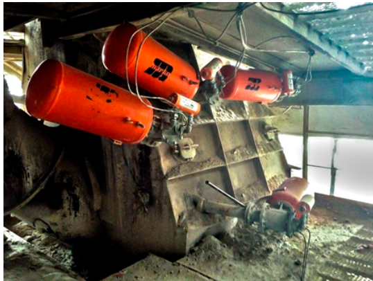
22 existing Martin® Tornado Air Cannons were upgraded with a Martin® Piston Return Reservoir to reduce operating costs.
