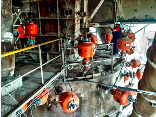
29 Hurricane Air Cannons supplied by Martin Engineering Turkey, each with a 70 liter reservoir, were installed in strategic locations.
