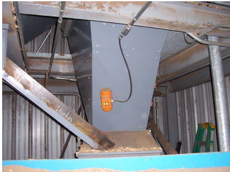
Photo: Martin Engineering. The brush cleaner is a unique electric-powered model that provides an effective, cost-efficient solution for residual belt-borne material. The secondary units are Martin SAF2™ Belt Cleaners, a versatile "deflected blade" design that features a gentle pressure to prolong service life and prevent belt damage.
