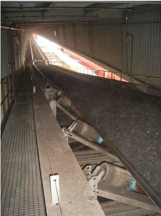
The terminal also anticipates as much as 40% longer belt life from the new chute design, as a result of reduced abrasion.
