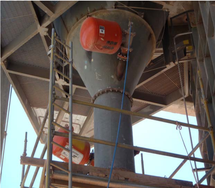
The original cannons were located in the entry to the kiln, cooler inlet and the preheater tower.
