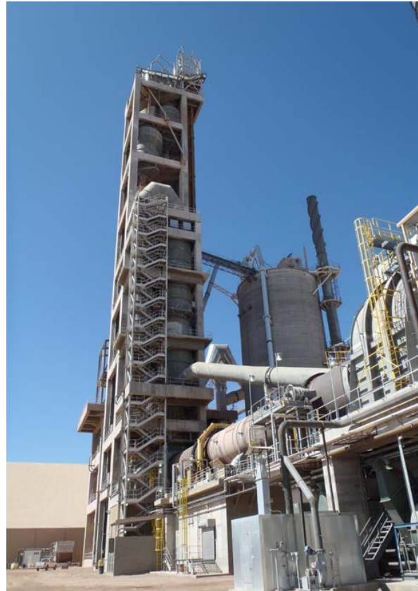
15 Air cannons from Martin Engineering were originally specified in critical locations, to control accumulation and enhance material flow.
