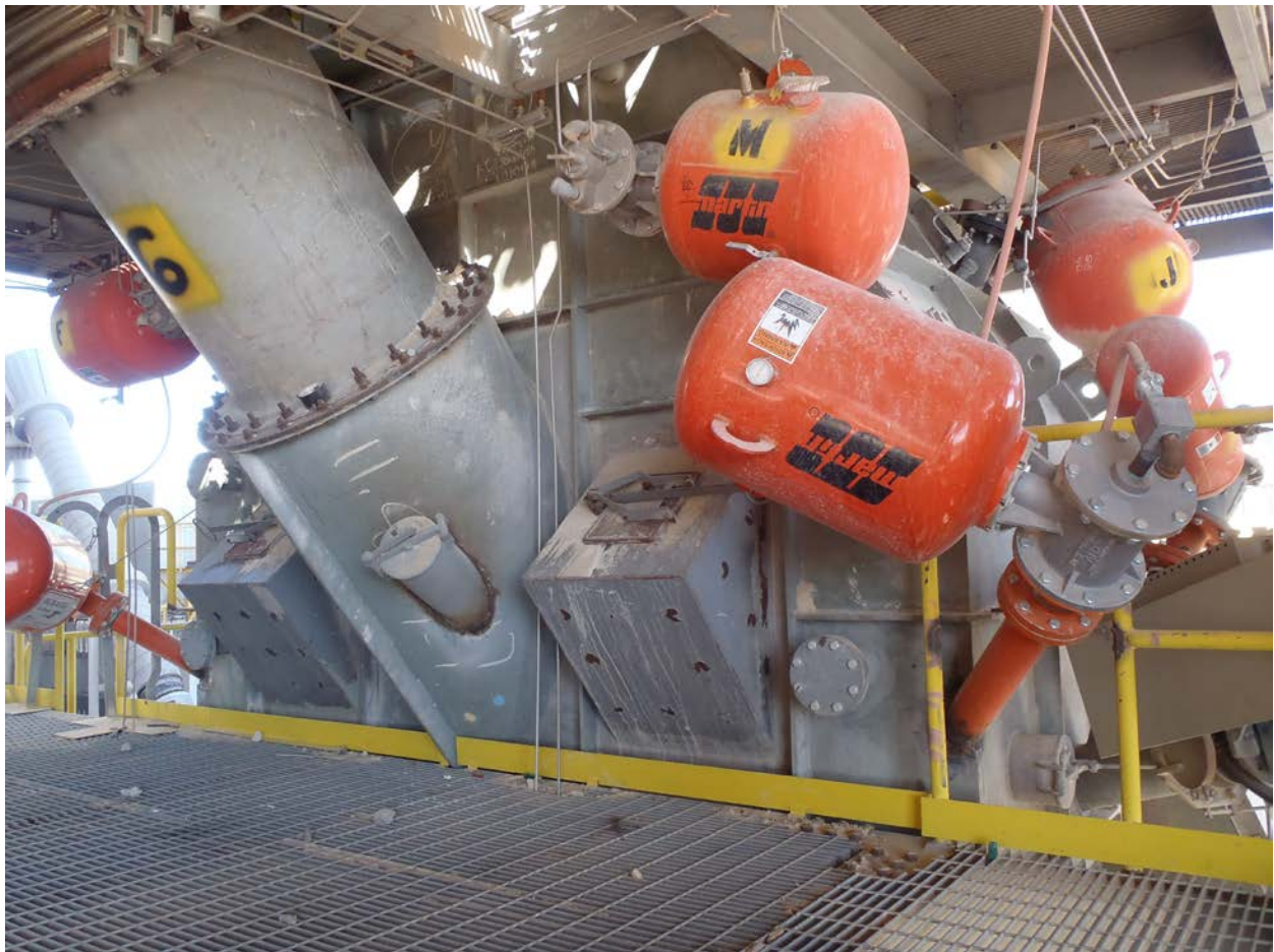
These cannons were positioned in the lower part of the pre-heat tower, near the automatic sampler.
