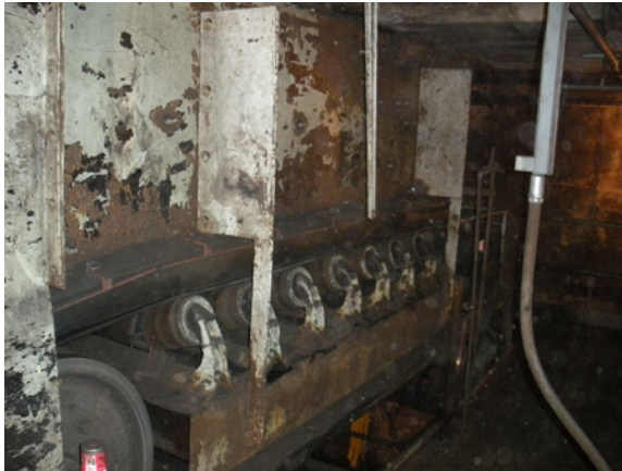
NIPSCO before: MCGS took a proactive approach to upgrading conveyor feed systems, conducting a plant-wide assessment and implementing a program designed to reduce fugitive dust and spillage.
