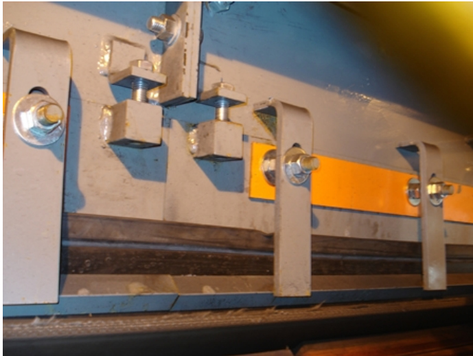
The wear liner is installed outside the transfer chutes, eliminating the need for confined space entry and avoiding a full tear-out of the existing chutes.
