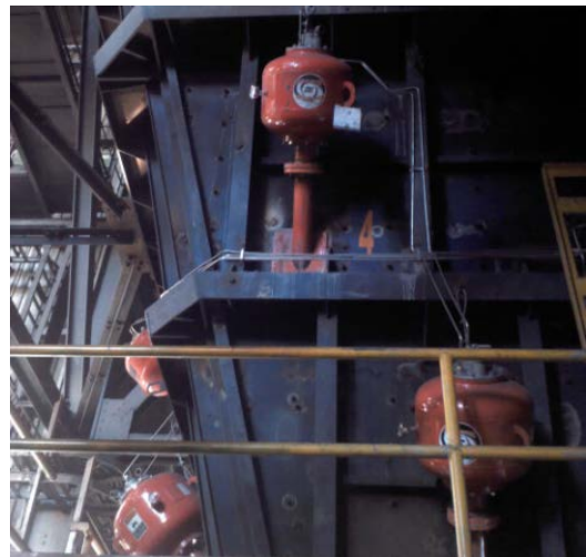
68 Martin® Air Cannons were installed on a total of 10 hoppers.
