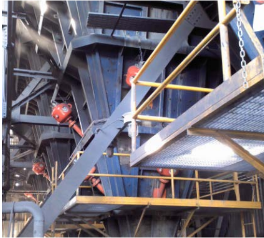
To minimize the blockage, the air cannons were installed in strategic points.
