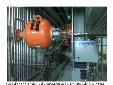
[Neponset, IL] – An innovative Minnesota energy company has eliminated labor-intensive air lancing to clean biomass ash from boiler walls by installing a series of high-powered air cannons to dislodge accumulations and restore process flow. The air cannon network at Koda Energy
