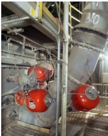
110 Martin® Hurricane Air Cannons are being installed in the two plants, covering preheater towers, additive silos and cyclones.
