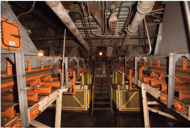
Martin Engineering upgraded four transfer points and twelve belts throughout the plant.
