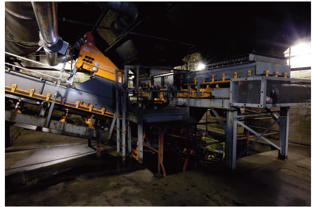
Insertable air cleaners were added to seven load zones to further reduce the escape of fugitive material.
