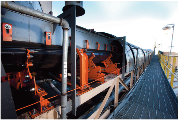
Transfer point upgrades aimed at combustible dust mediation were needed to improve the overall safety of the plant.
