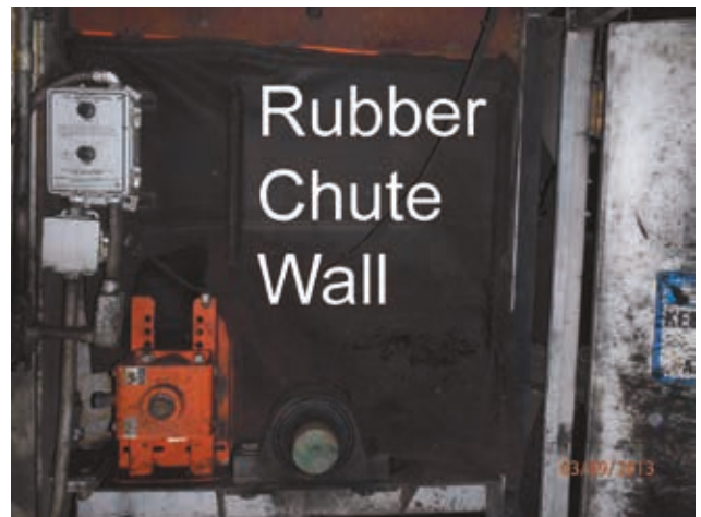
Figure 6. Rubber chute wall seal.
