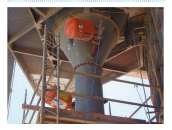
technology has developed a proven track record around the world for relieving bulk material bottlenecks. The Martin<sup>®</sup> XHV Air Cannons, which were installed when the plant was built, fire a powerful discharge of compressed air to remove material adhered to the vessel walls.
